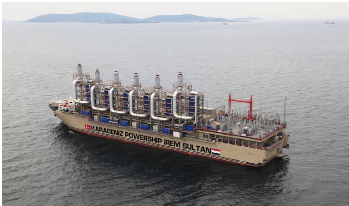
Power ship with MAN 51/60DF engines and heat recovery steam turbines with total power >110MW
